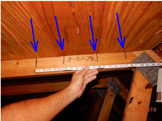
#21 8 D Nails Spaced 6" OC
