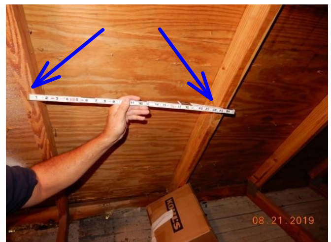
#18 Trusses Spaced 24" OC
